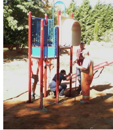
No. 6 Mine Playground Equipment Installation
